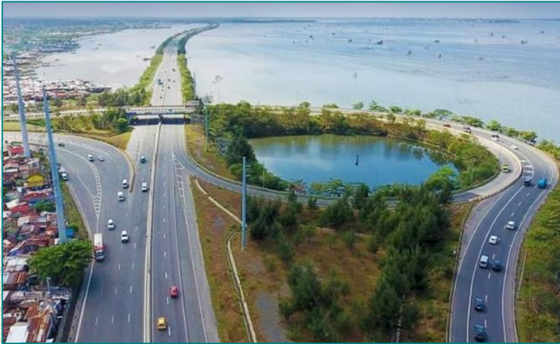
CAVITEX (Cavite Expressway)
